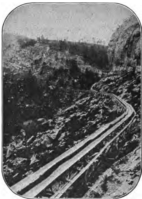
FIG. 122.—V-shaped board flume floating sawed lumber out of impassable Rocky Mts., Canyon, Wyoming. At the right center a creek adds to the water supply. At the right of the flume is a running board for workmen. (U. S. Forest Service.)
